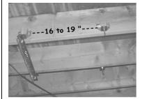
• Step # 4: Slide the UFS subwoofer, foam side up, into place and install second angle iron as above. Tighten all 4 nuts progressively until the front side foam compresses about 1/8".
